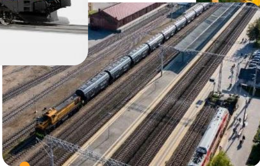
Construction of a repair depot in Vaidotai
